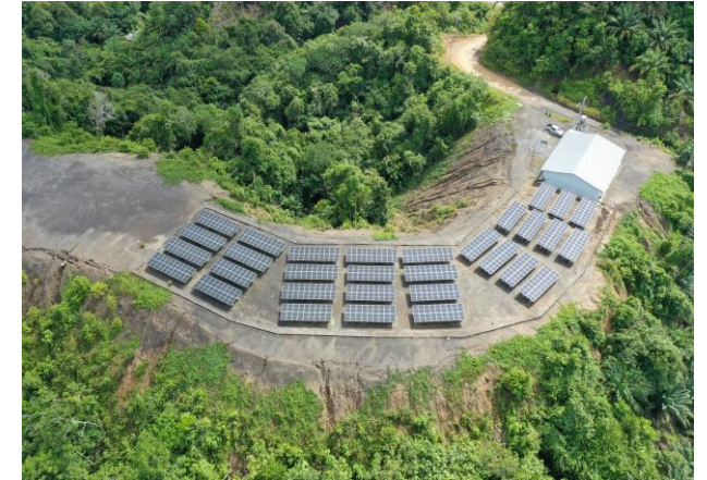
(Mini-red fotovoltaica © Sarawak Energy Berhad)
